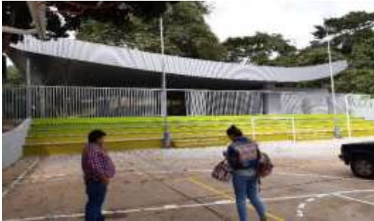
VISTA GENERAL AREA INTERVENIDA
